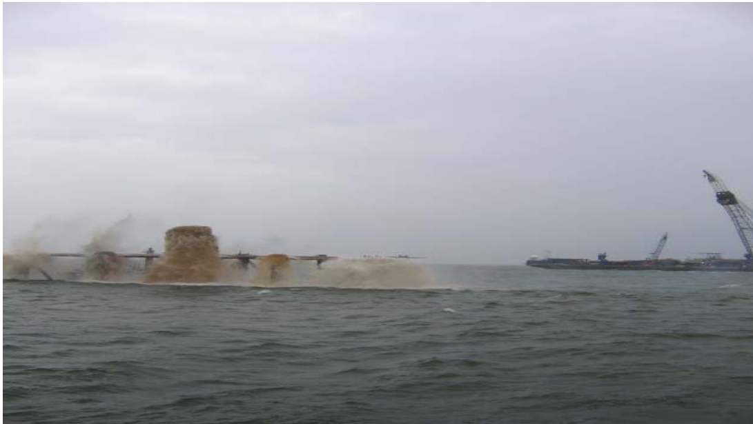
Photo #7: Delay shot sequence on piles A1 through A5 and B1 through B5 and conductor F3
