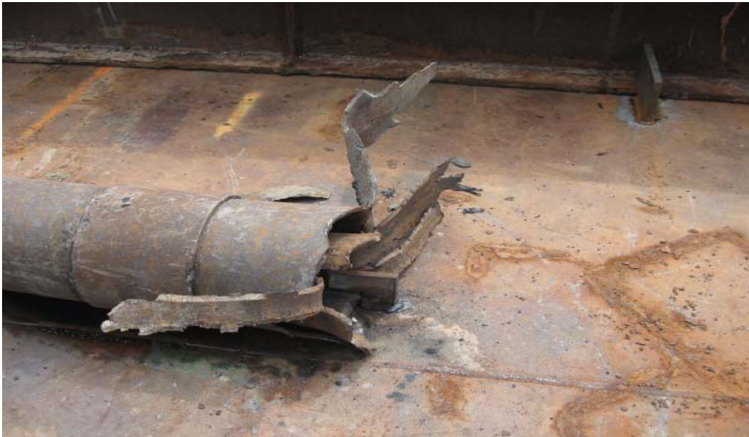
Photo #3: Conductor Severed with 50 Pound Bulk Charge (Shot Sequence #1, but Typical of Bulk Charge Cut)
