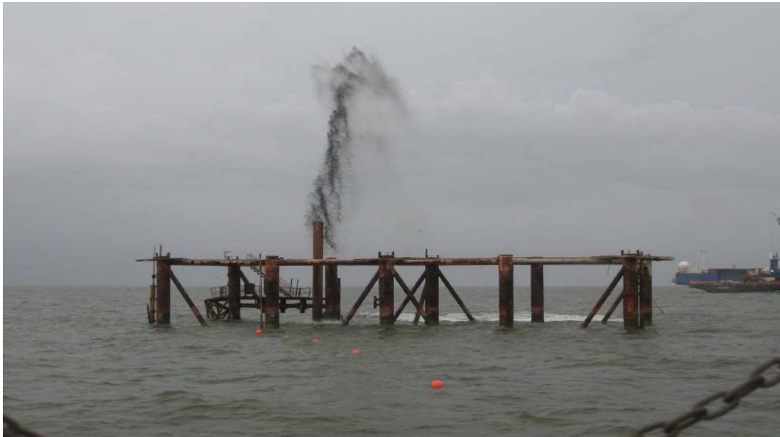
Photo #5: 50 Pound Bulk Charge Shot on Conductor Internal to Structure-- Array Buoys in Foreground (First Shot Unsuccessful). Shot Sequence #3.
