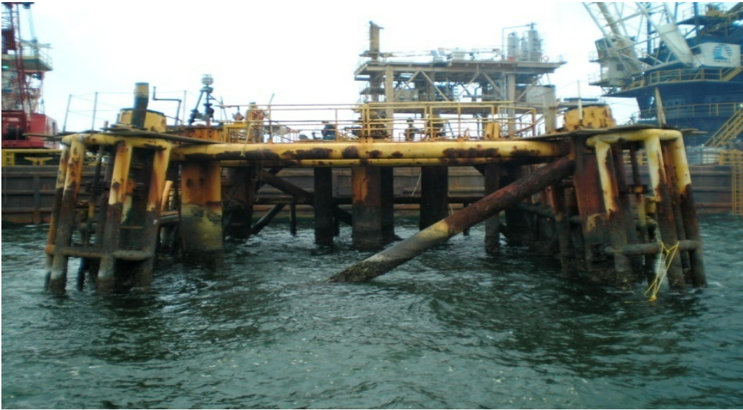
Photo #9: Merit EC-32 A Platform Structure
