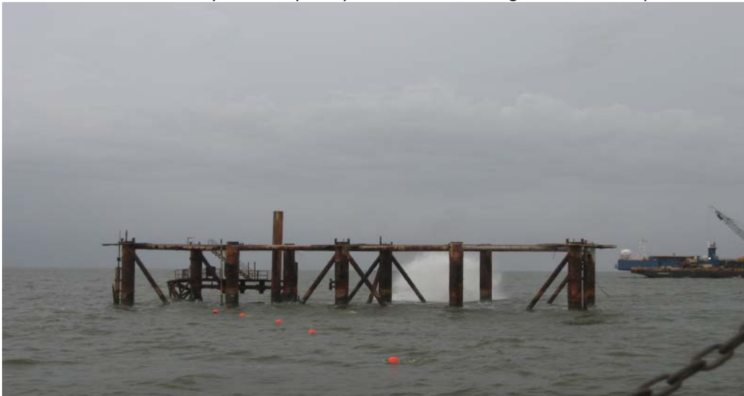
Photo #4: 75 Pound Bulk Charge Shot on Caisson Sub-sea Stub Diver Cut 4ft ABL (shot Sequence #2)
