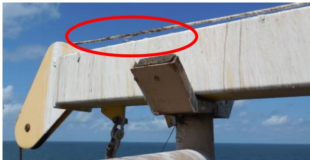
Figure 1 – Corroded crane cable
