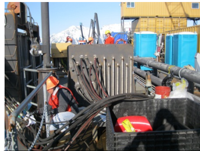
LSC-5 Hydraulic Control Panel
