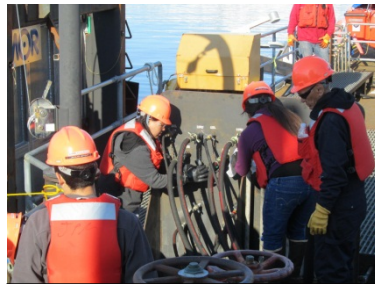
Assembling Power Pack
