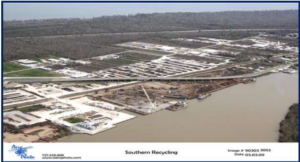
Figure 8-1. Southern Scrap Yard Morgan City
