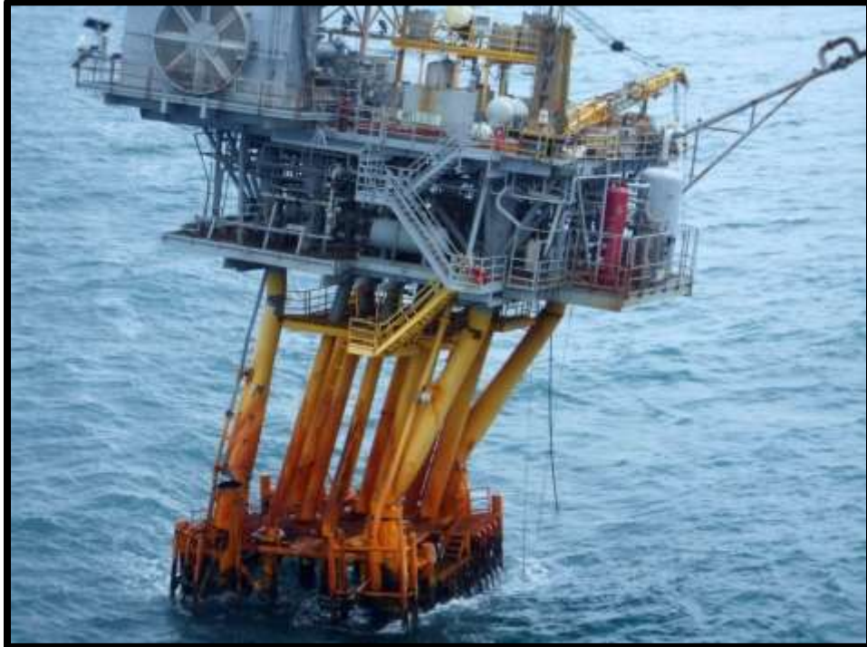
Figure 5-11. Hurricane Ike Damaged Platform, 2008
