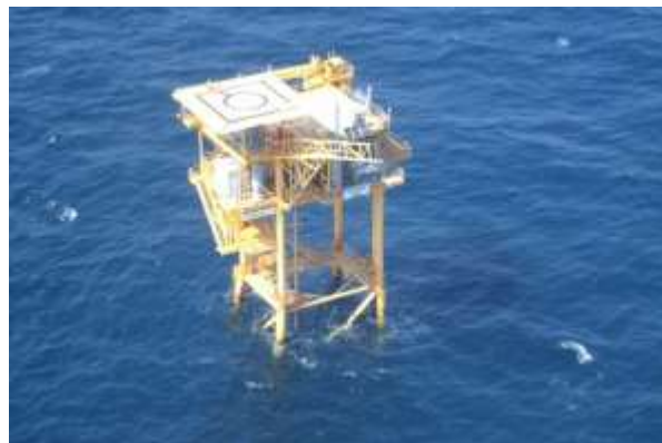
Figure 3-14. 4-Pile Well Protector
