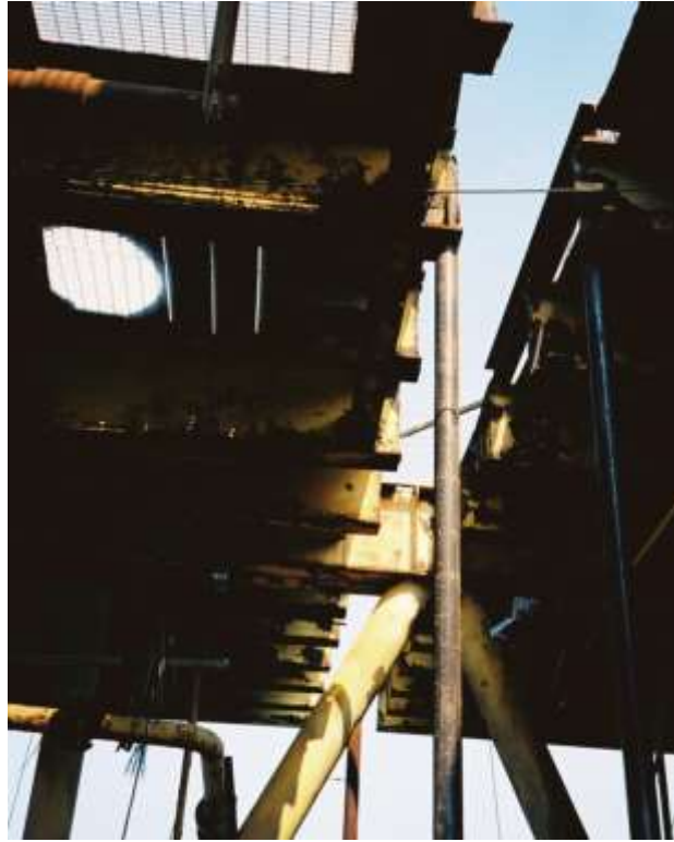
Figure 5-7. Deck Severed into Lift Sections
