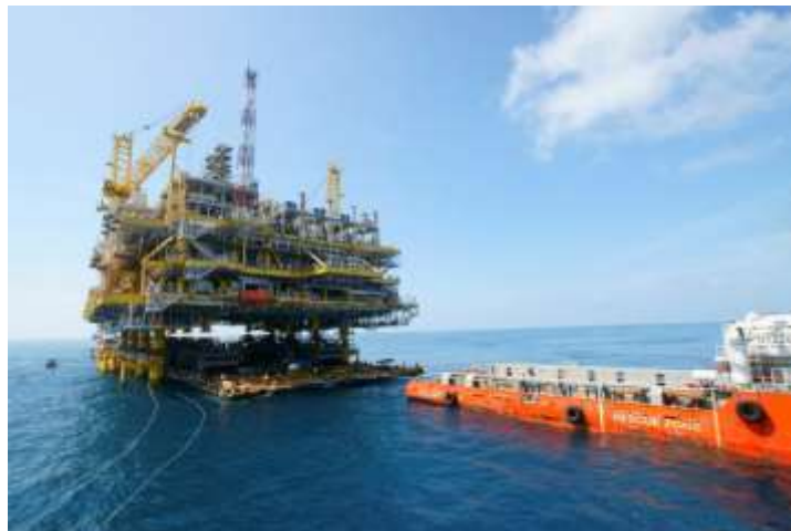
Figure 4-1. Deck Ready to Be Installed
