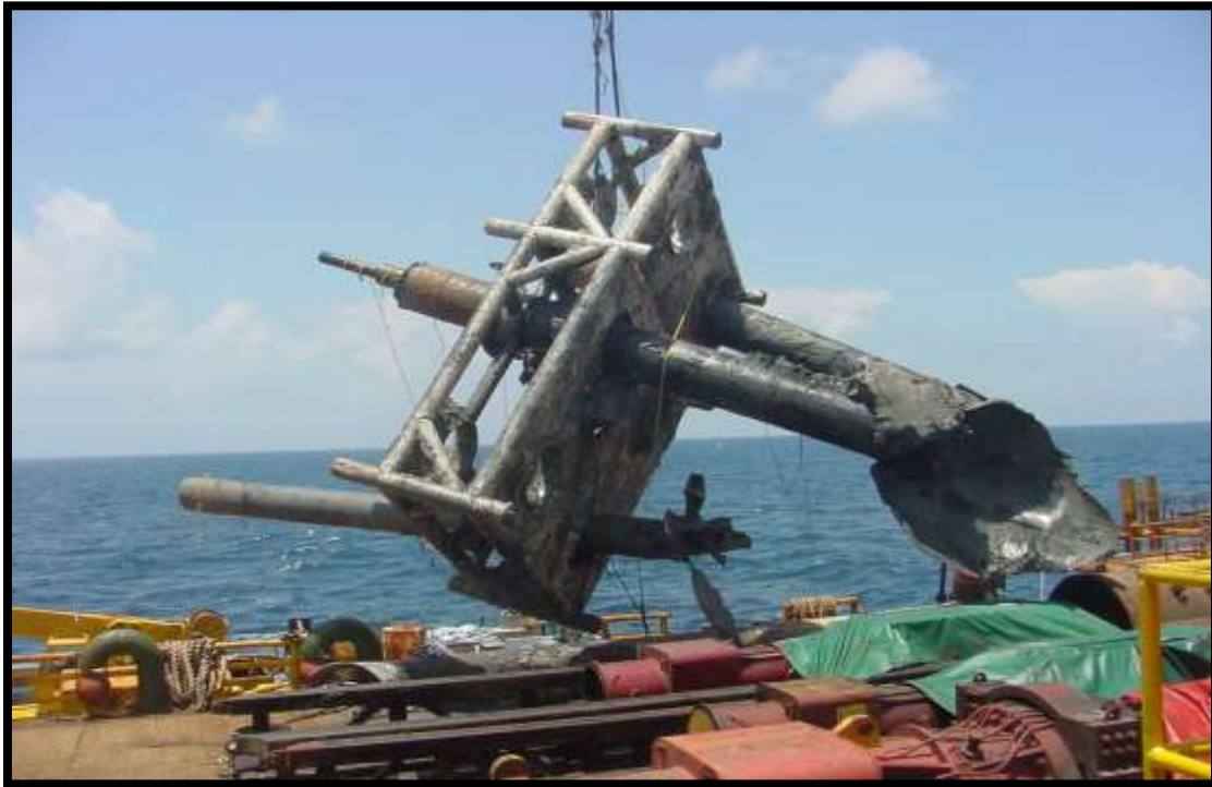
Figure 6-13. Template removal by explosives (Photo courtesy of Demex International)
