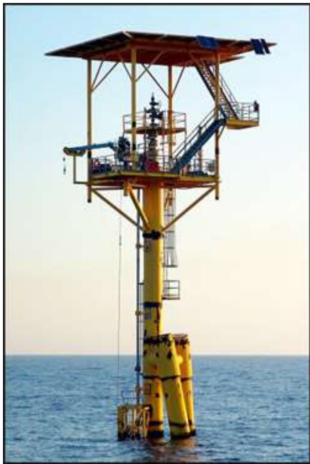
Figure 3-2. Typical Caisson Platform Components
