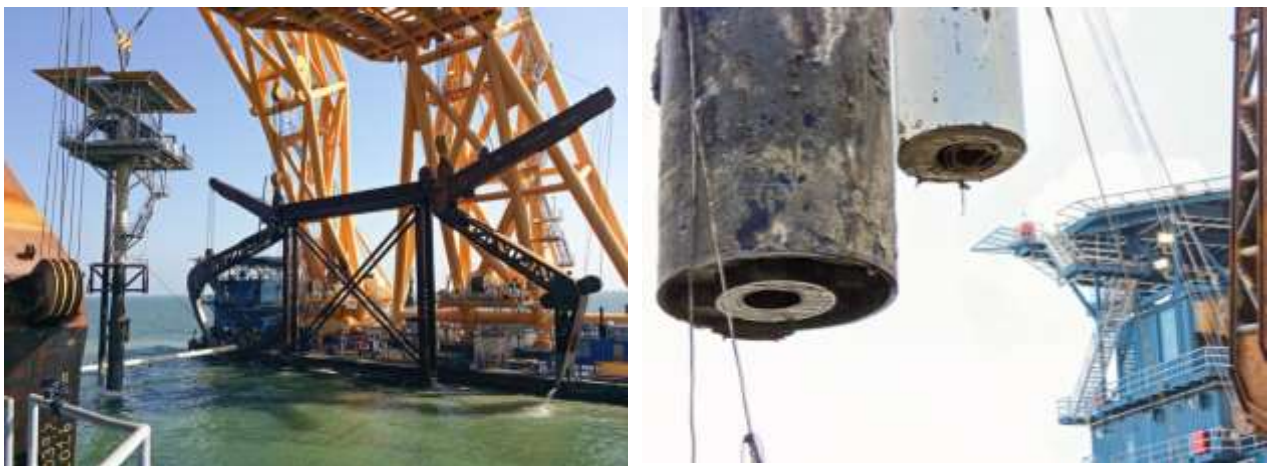
Figure 6-28. Grouted Caisson Severed with Tungsten Beaded Wire
