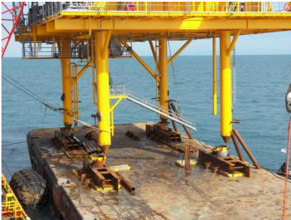
Figure 5-8. Setting Deck for Seafastening
