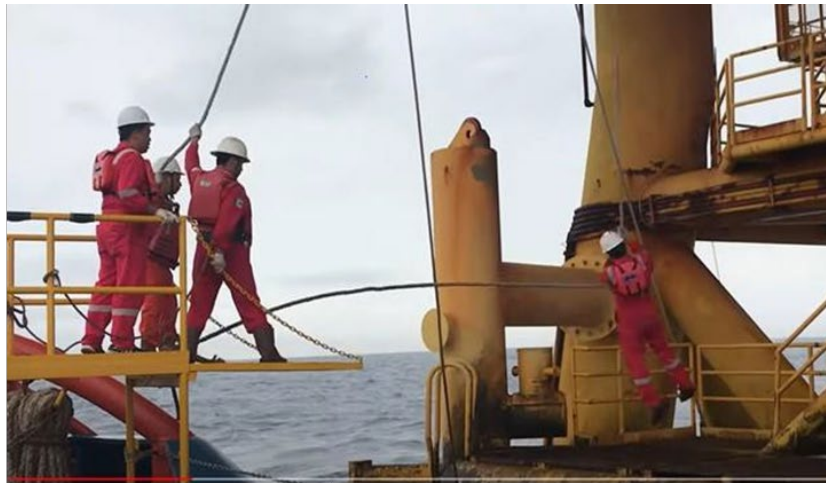
Elevated Platform Structure.
