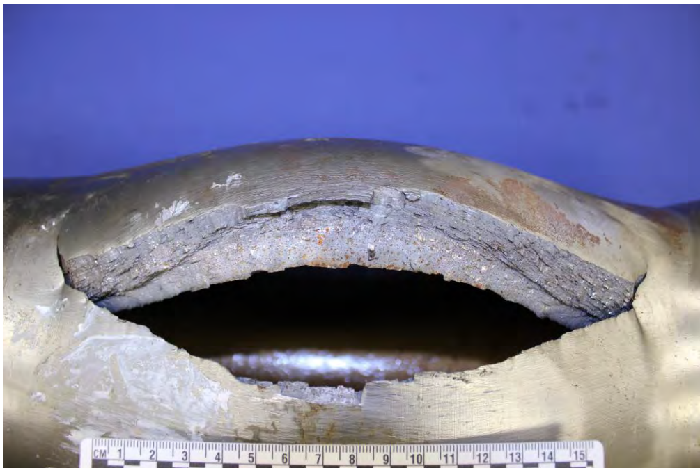
Figure 4: As Received Photograph – Sample 2 – Close-up View at Burst (scale in mm)
