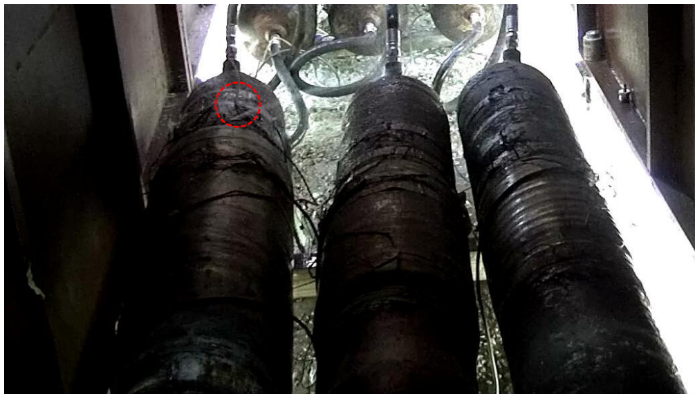
Figure 4-10: Photograph of failure (circled) during cycling of Manufacturer A’s Tension sample.
