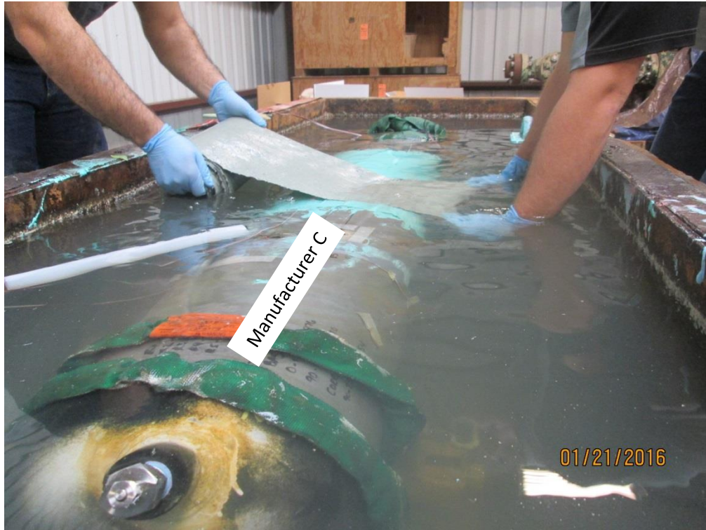
Figure B-11: Manufacturer C repair installation (3 of 4)
