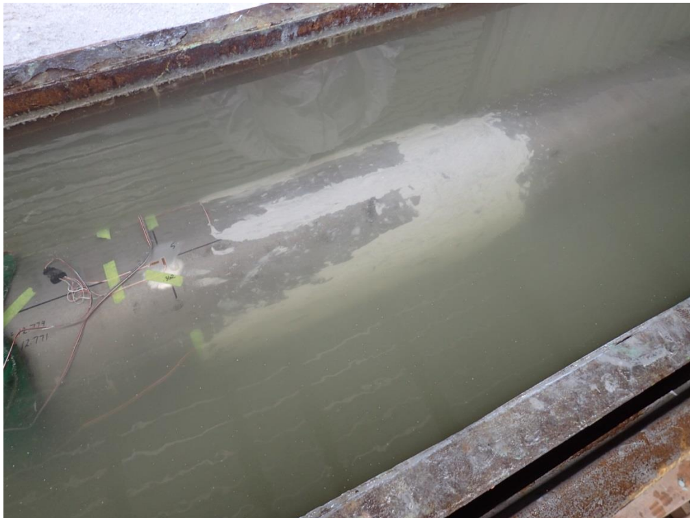
Figure B-4: Manufacturer A repair installation (4 of 4)
