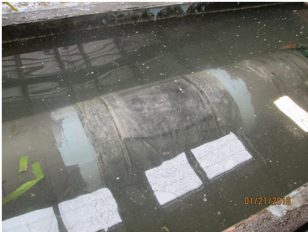
Figure B-8: Manufacturer B repair installation (4 of 4)
