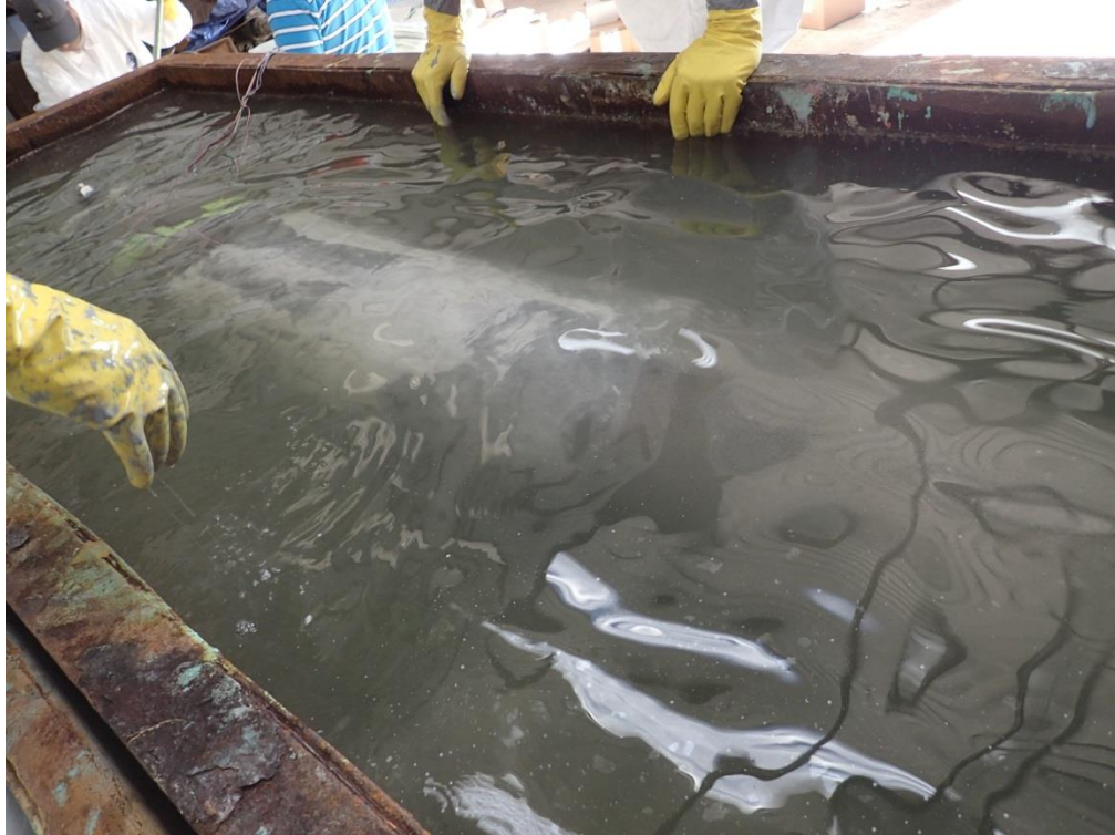
Figure B-2: Manufacturer A repair installation (2 of 4)
