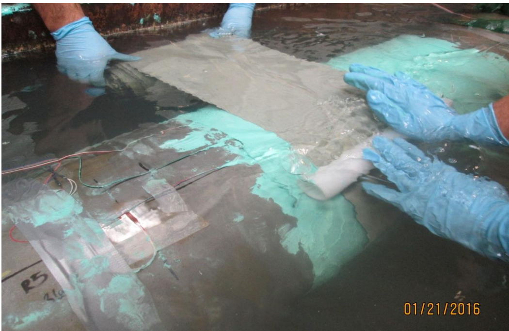
Figure 3-5: Representative photograph during installation of Manufacturer C's repair.
