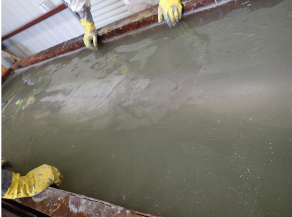
Figure B-3: Manufacturer A repair installation (3 of 4)
