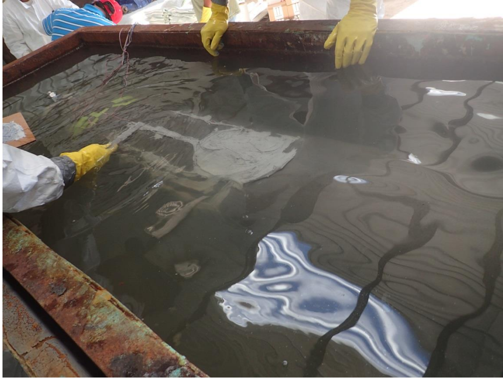
Figure B-1: Manufacturer A repair installation (1 of 4)
