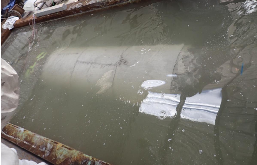
Figure 3-4: Representative photograph during installation of Manufacturer A's repair.
