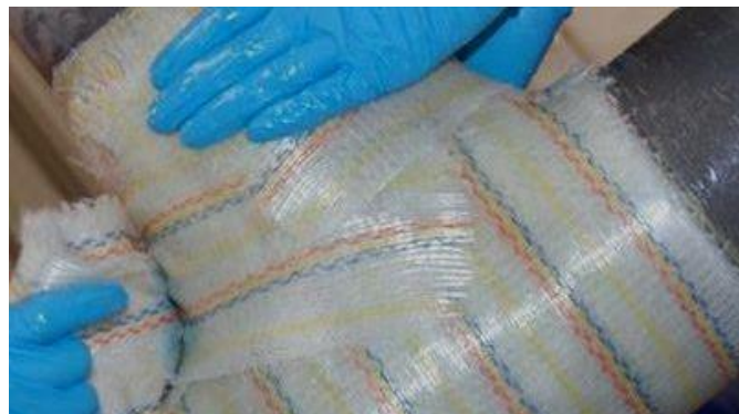
Figure 1. Application of a Technowrap 2K composite repair.
