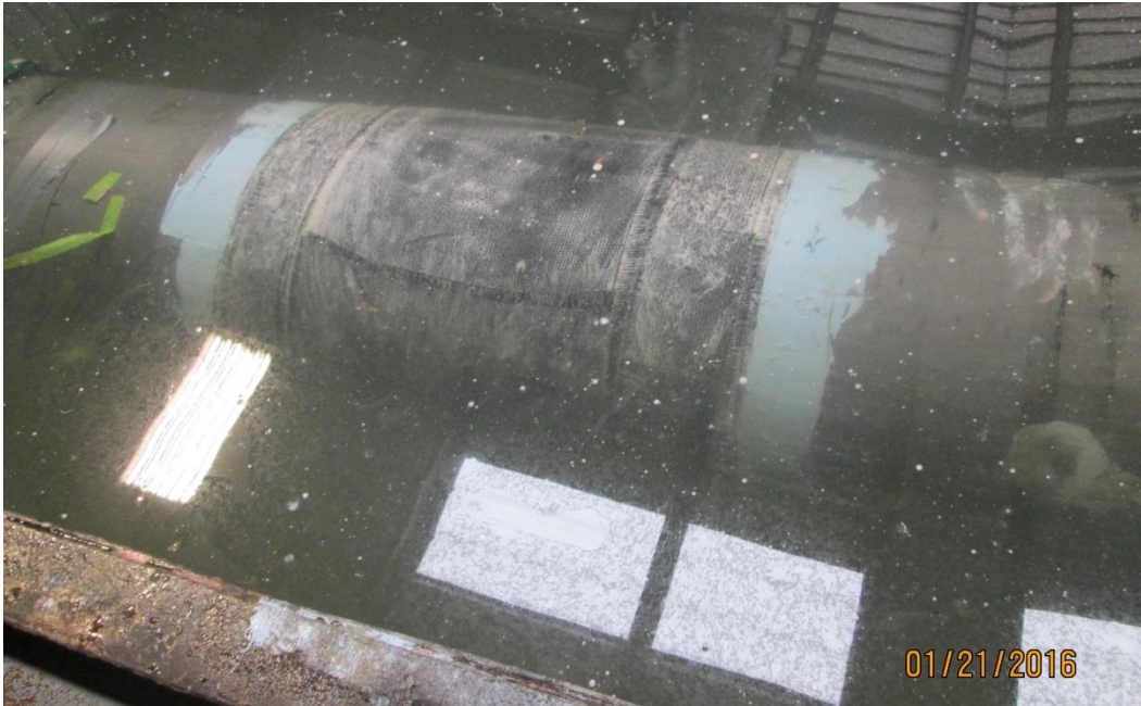
Figure 3-6: Representative photograph during installation of Manufacturer B's repair.
