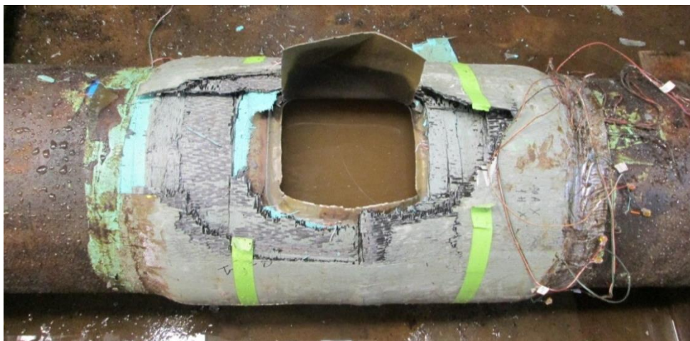
Figure 5-5: Manufacturer C’s burst sample post-test – failure in simulated corrosion region
