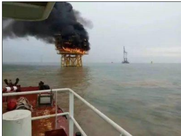
Figure 3 – SPIC Binhai North offshore substation fire [10]
