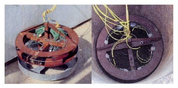
FIGURE A-7 LSC delivery system with retracted casings (left) and a similar design being lowered into a pile (image courtesy of Explosive Services International; Saint-Arnaud et al. 2004)
