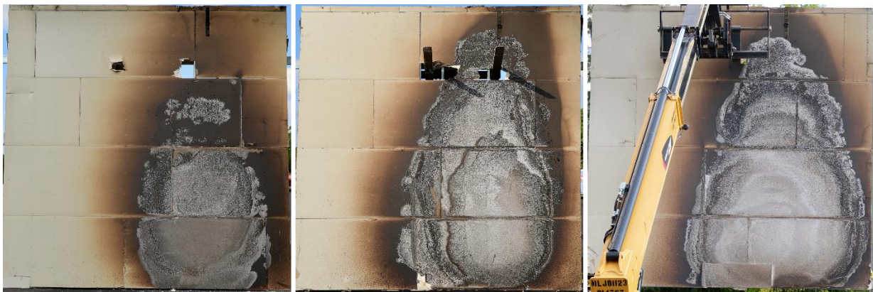
Fig. 48 Photos of the walls after experiments
