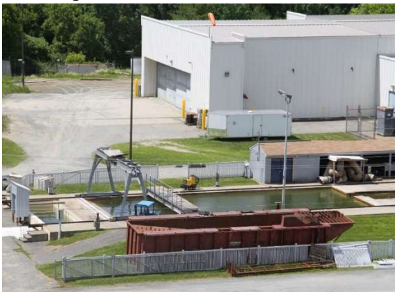
Figure 2-1. Geophysical Research Facility at CRREL - 20m x 6.7m x 2.1m; water-filled tank.
