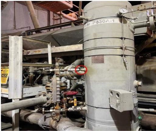
Figure 2-Photo shows 3/4-inch unsupported pipe nipple on suction scrubber.
