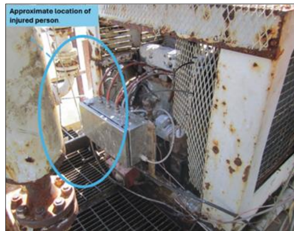
Figure 2: Position of an injured worker during time of incident. The worker was adjacent to the engine observing the magneto while another worker operated the start valve. (Incident 1)
