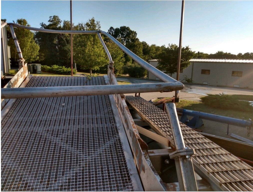
Fig. 21 Photo of damaged canopy frame.
