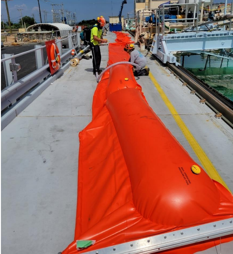
Fig. 3 Elastec Airmax half-size boom.
