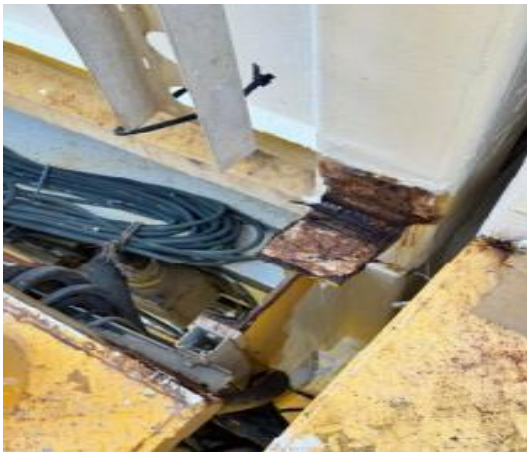
Walkway separated outward from temporary living quarters, exposing a significant gap.
