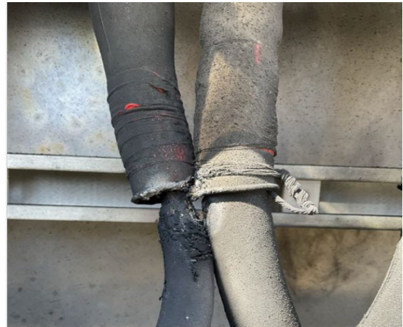
Figure 2: Burned wiring located below the stress cones between the line and load conductors.
