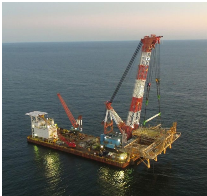
Figure 10-1 – Heavy Lift Vessel DB Thor
