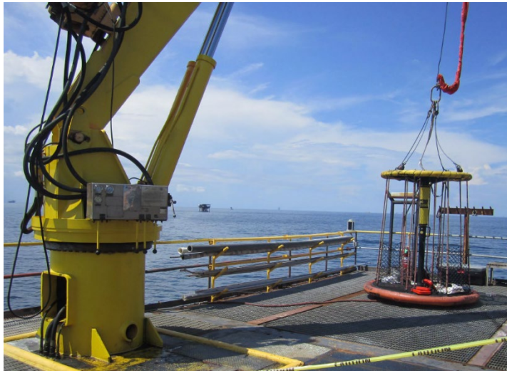
Figure 1: (Incident 1) Crane and personnel basket type involved in incident.
