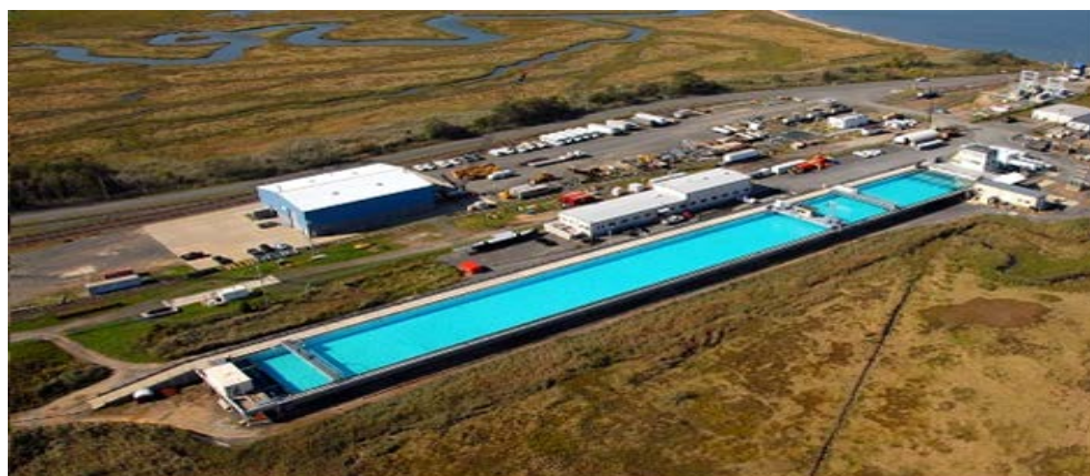
Figure 2: Ohmsett Facility in New Jersey
