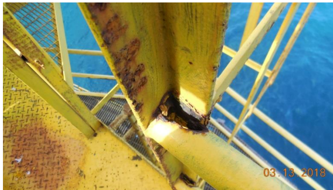
Handrails near the top of the crane access ladder corroded
