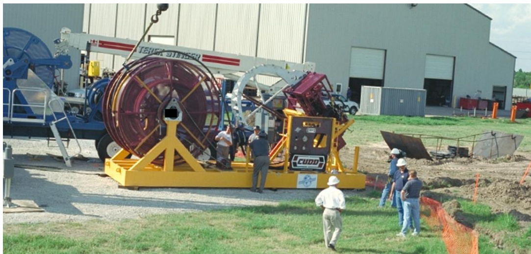
Figure 65. Subsea Horizontal Coil Tubing Unit
