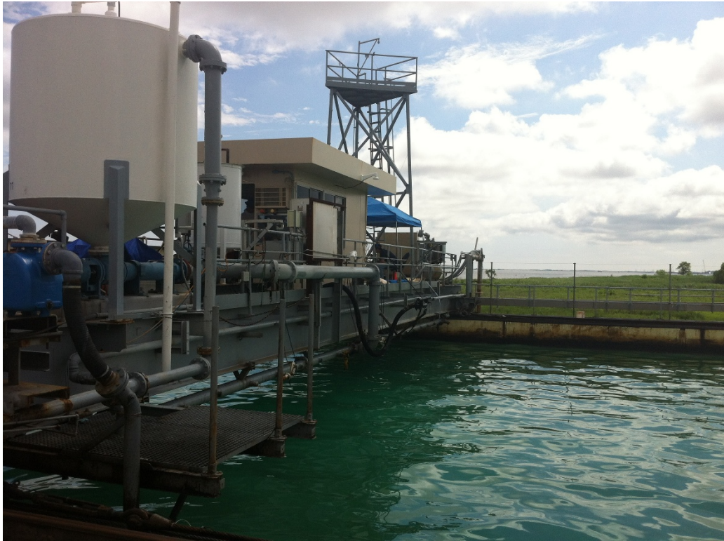
Figure 29. Ohmsett control room bridge and oil distribution system.
