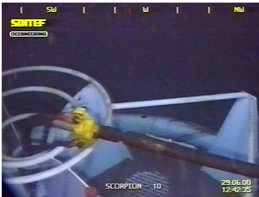
Figure 7.3. Picture identity 12-42-35. A switch is made to color camera for a closer look at the leakage point.
