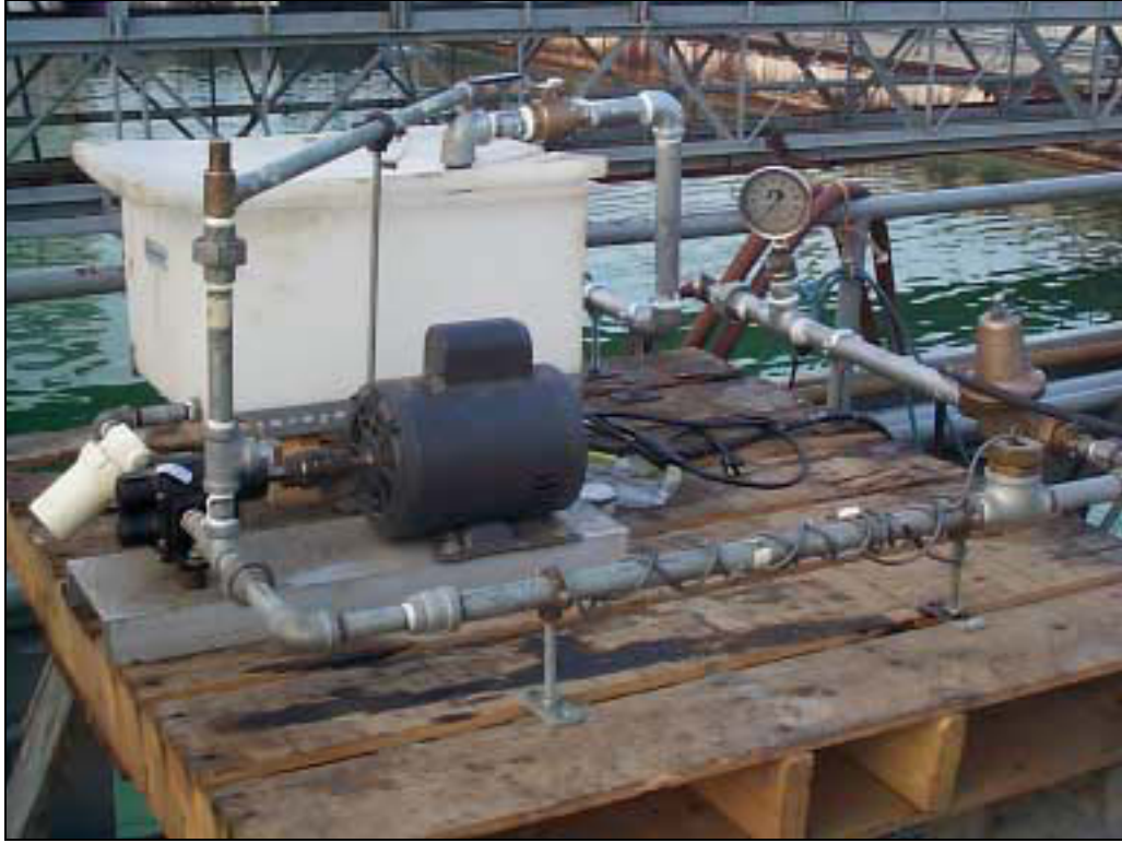
Figure 7. Dispersant Supply Tank and Pump
