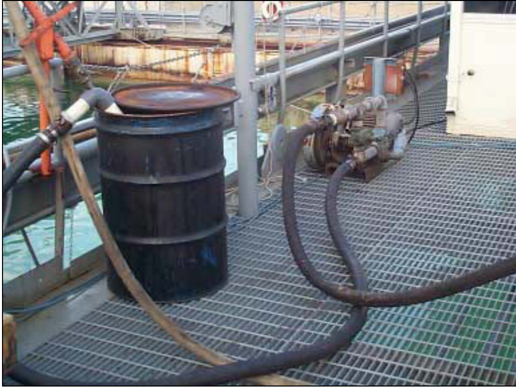
Figure 6. Oil Delivery Pump and Supply Drum
