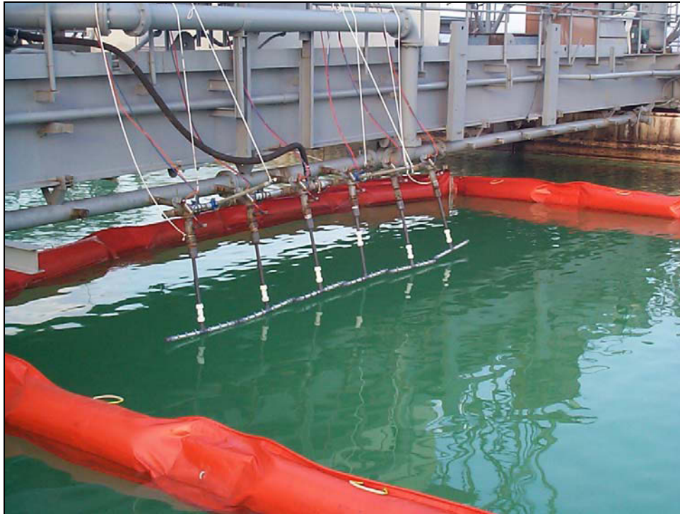
Figure 2-2: Oil Distribution System, October 2003.
