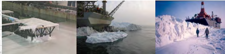
Ice rubble formation on gravity based structures (D-6, Prirazlomnoye, SSDC) and a SPAR.
