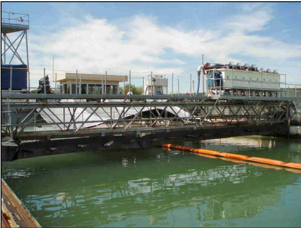
Figure 3. Boom was placed down the water surface
