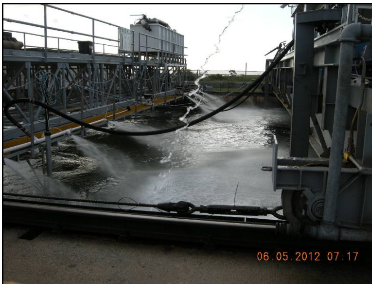
Figure 2. Oil Movement Spray Jet System
