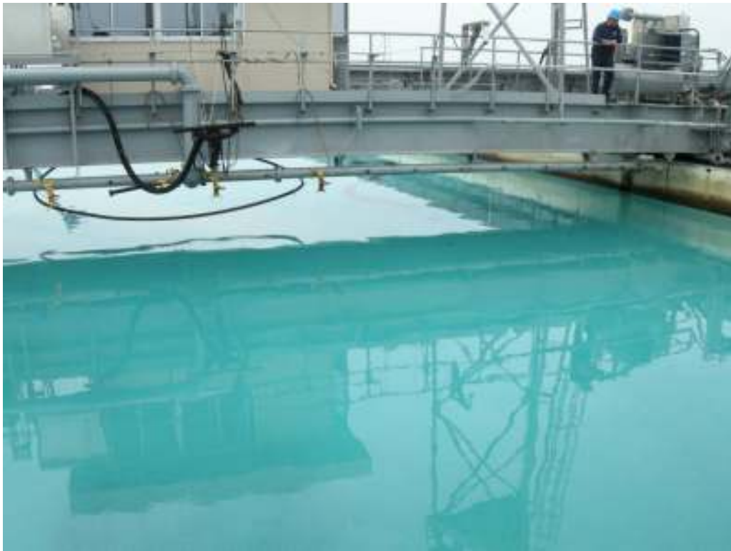
Figure 17. Containment ring lifted up and secured under Main Bridge.
