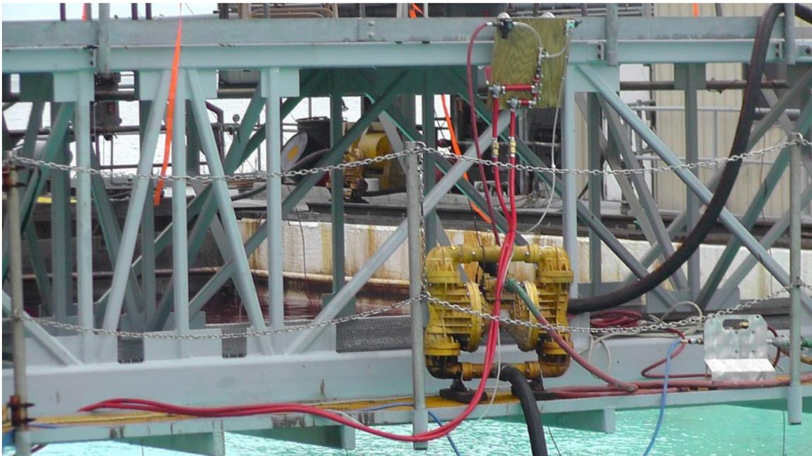
**Figure 15:** Location of double diaphragm air pump (yellow) and air manifold board (above yellow pump with red air lines) on the Auxiliary bridge.
