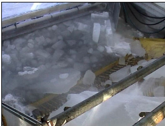
A lot of broken ice and slush encountering the Lifting Grated Belt.
