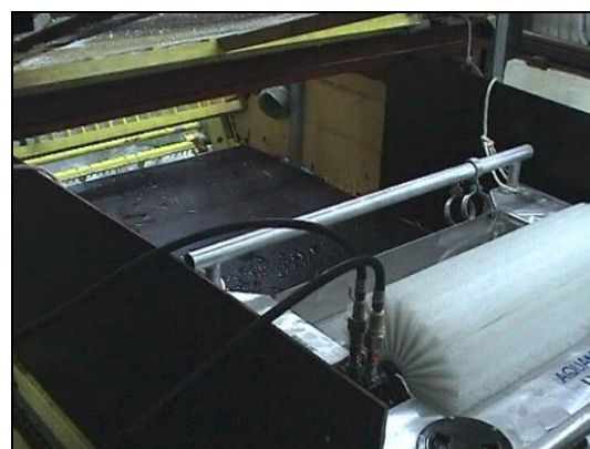
Modified Aquaguard RBS-10 installed inside LGB prior to testing.
