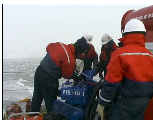
Priming the pump for the water flushing.
