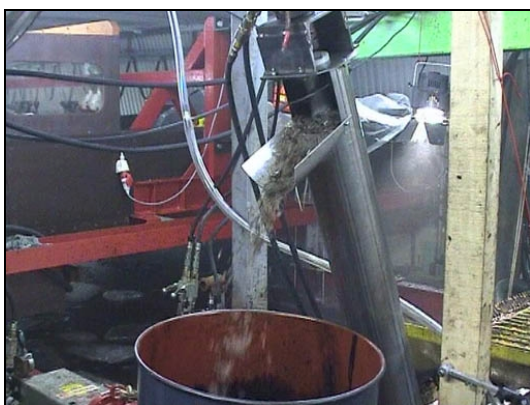
LORI brush unit after installing augers for transfer of recovered product from the rear trough. We see oil and ice being transferred to the open top container.
