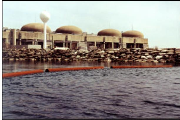
**Figure 2.7: Ice Boom Deployed at the Pickering Nuclear Generating Station Ice Boom, in February 1999**
