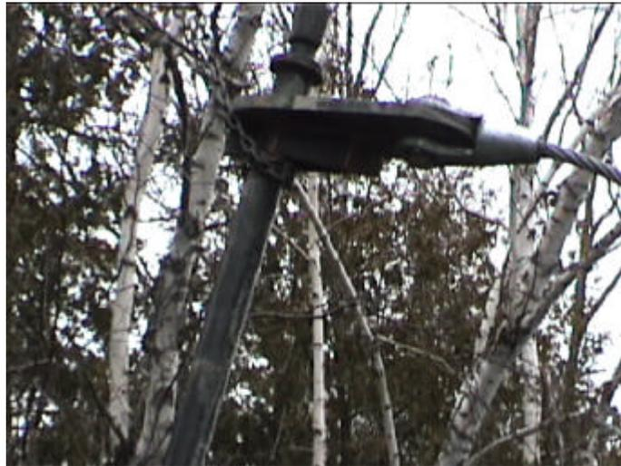
**Figure 5.10: Anchor Used for Rock Bottoms**
