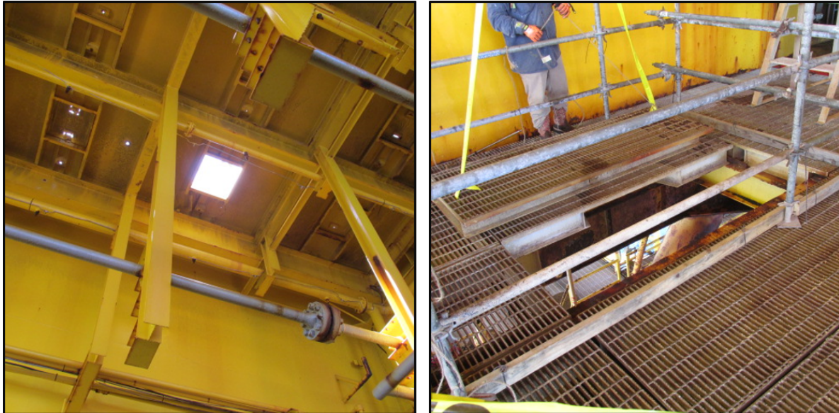
Figure 5 – Lowering the grating
