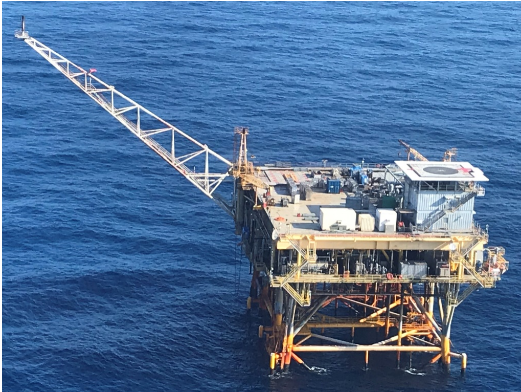
Figure 2 – Ewing Bank Block 826 Platform A
