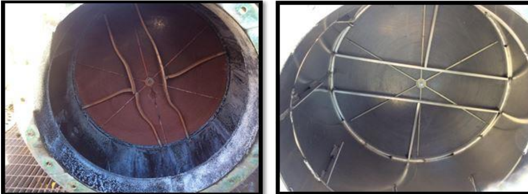
Figure 22: Existing Spark Arrestor (left), Compared to New Spark Arrestor (right)
