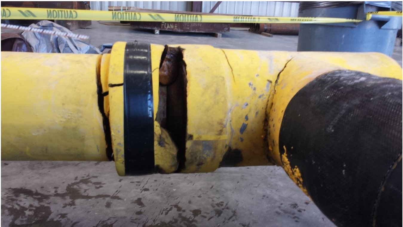
Figure 7 Load Limiting Joint Fracture
