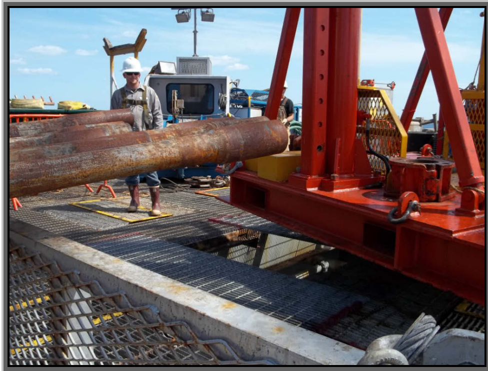
Figure 29 – Reenactment: PS & “pipe rack” obstruction during lift (three)
