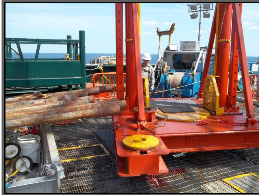
Figure 28 – Reenactment: PS & “pipe rack” obstruction during lift (two)
