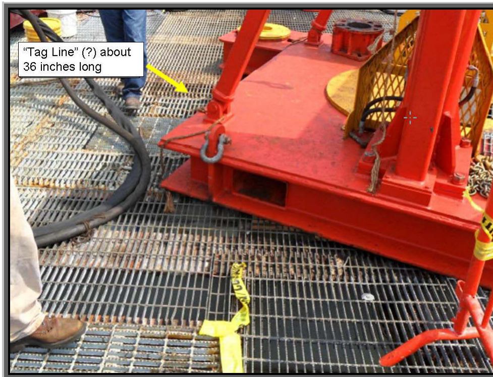
Figure 14 – Original tag lines on power swivel, Flagman corner
