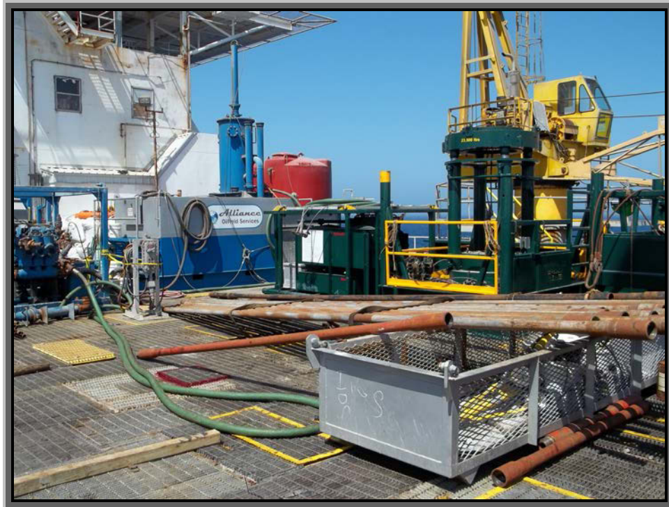
Figure 17 – “Pipe rack” and equipment on main deck
