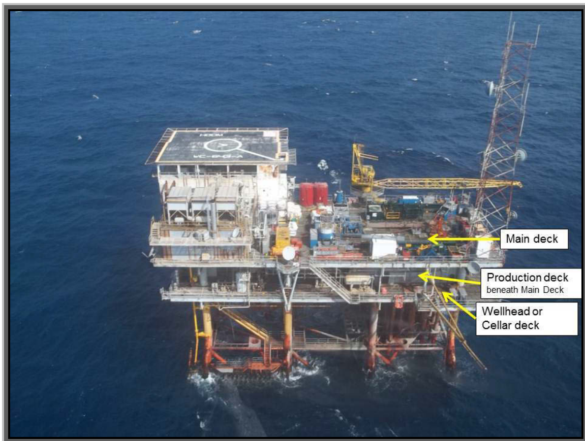
Figure 2 – West Cameron, Block 643, Platform A
