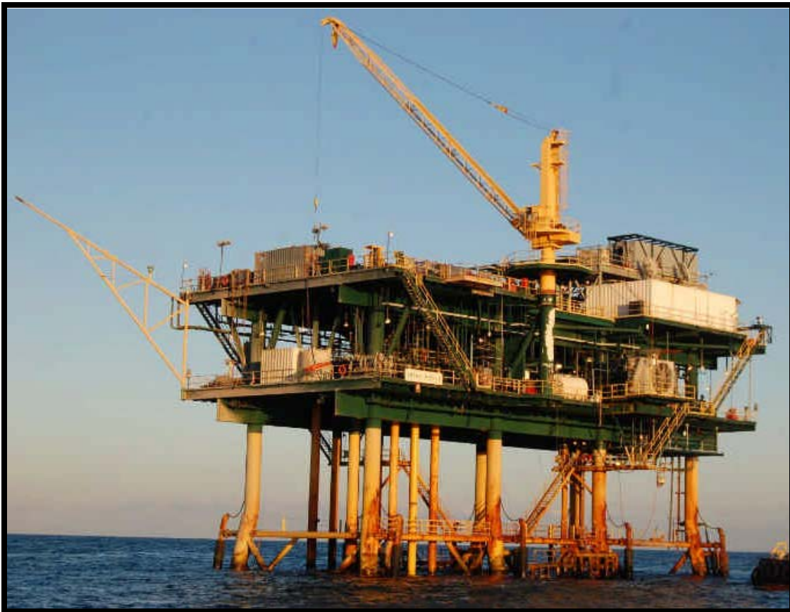
Figure 3 - HI A557 "A" Platform
