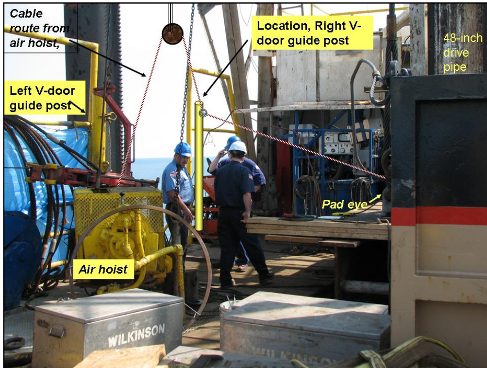
Figure 3: Method of rigging up to rotate 48-in drive pipe
