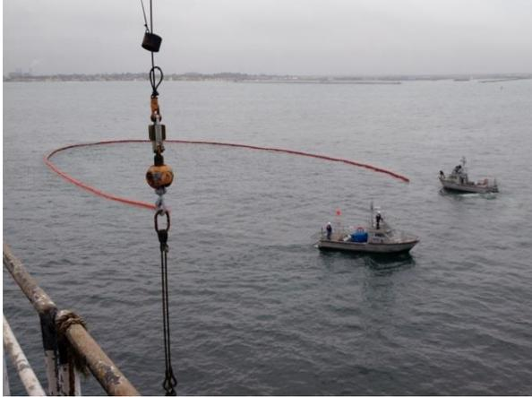
*Figure 2.* Small boats deploying containment boom near a facility using the U-shaped boom configuration (Source: BSEE).
