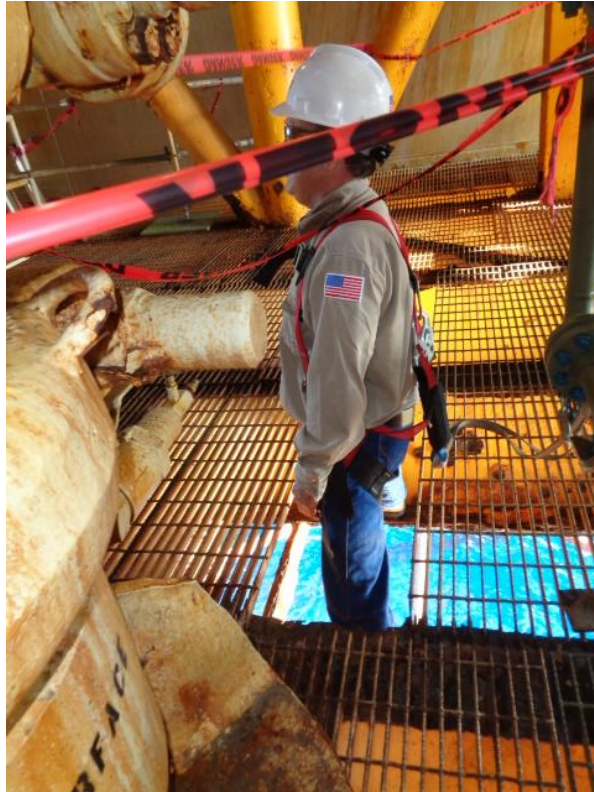
Figure 9- Post-Incident Photograph of the Production Superintendent Wearing Fall Protection Standing in the Open Hole After the Hazardous Grating Section was Removed
