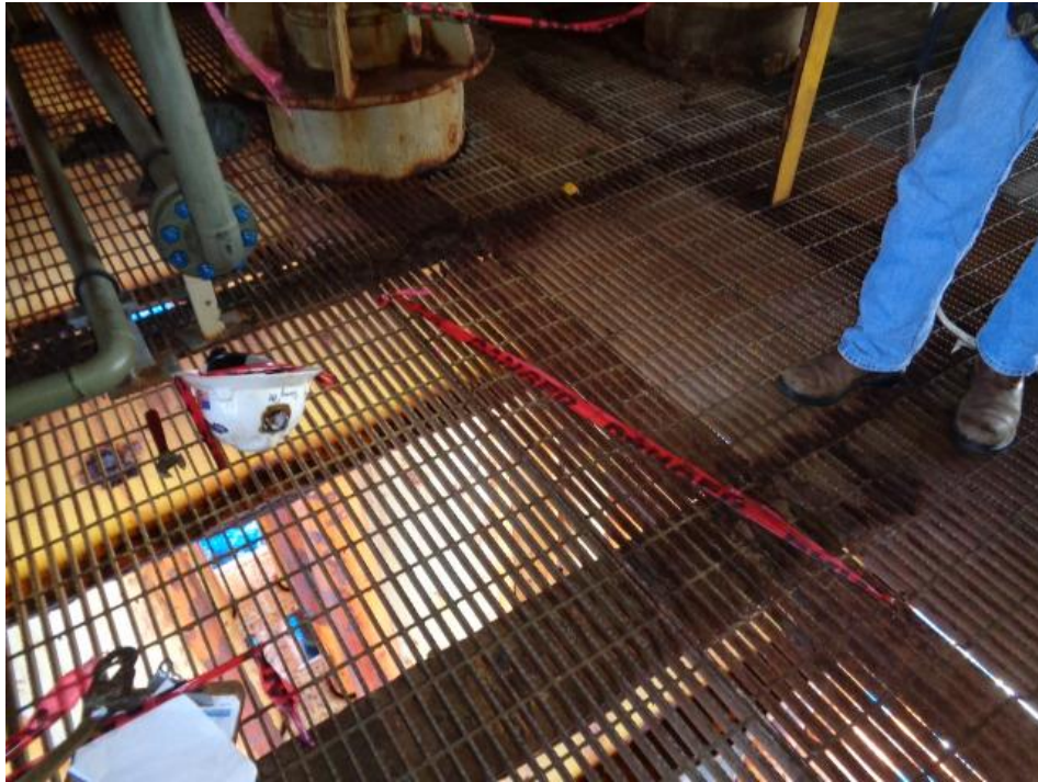
Figure 11- Post-Incident Photograph of Hazardous Grating Section Placed in its Approximate Pre-Incident Position
