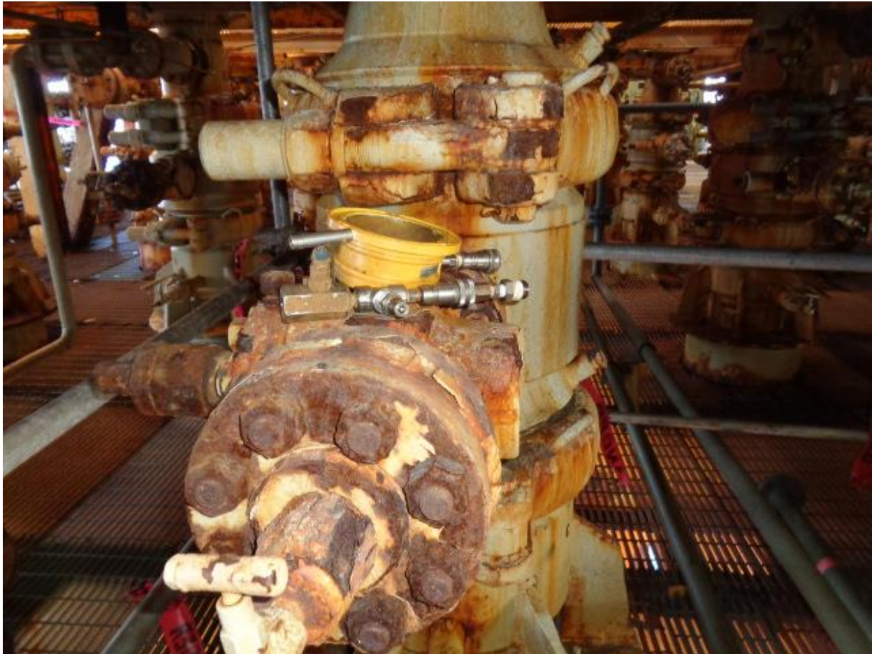
Figure 16- Post-Incident Photograph showing the Location of the Pressure Gauge and Testing Manifold on Well B-16
