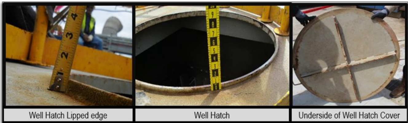
Figure 8: hatches and hatch cover (June 4, 2019)
