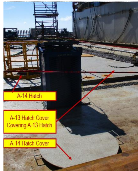
Figure 11: View of Well Bay Area from approximate location of A-14 Hatch Cover (June 4, 2019)
