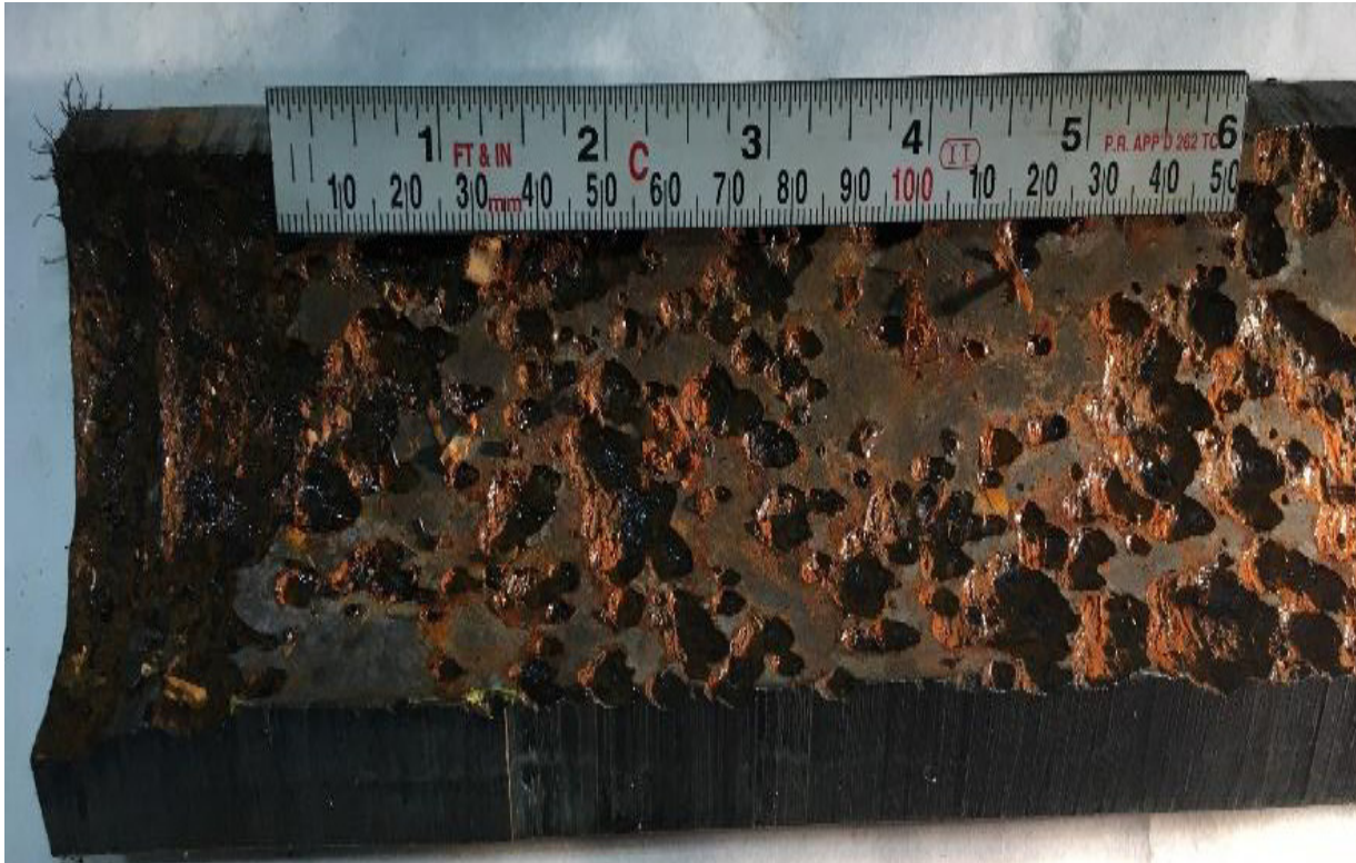
Figure 7- Pitting on inside of jumper
