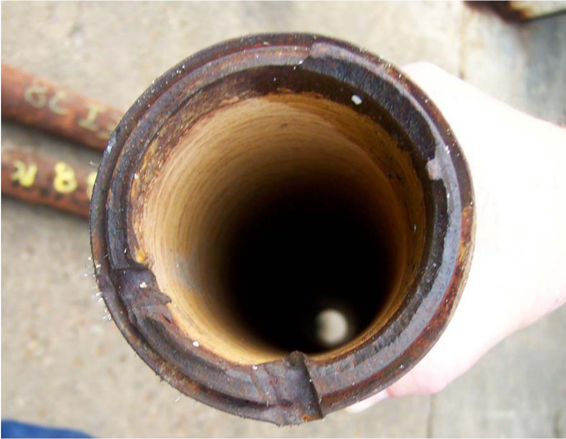
Photomicrograph showing the failure surface of the first failed tube prior to cleaning. Note the deep indentations most likely the caused by the fishing operation.
