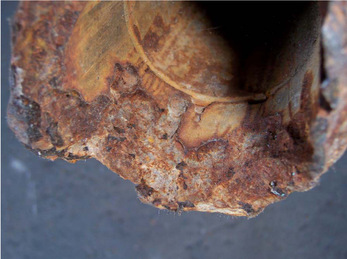
Photomicrograph showing the fracture surface of Piece#2. Note the extreme flow cut areas which caused extreme wall thinning. This would also greatly reduce the load carrying capacity of the tubing.
