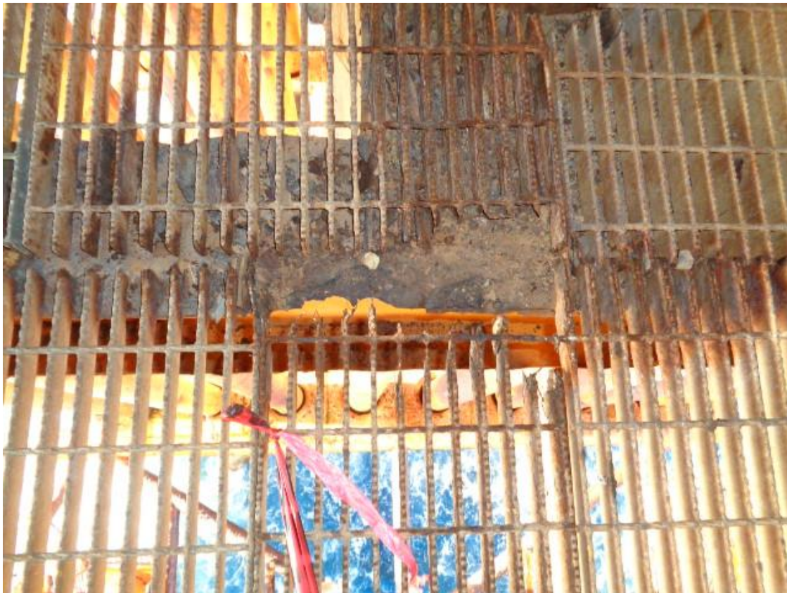
Figure 6- Pre-Incident Photograph of Hazardous Grating Section with Red Danger Marking Tape Affixed and After Impact from Sledgehammer Strikes
