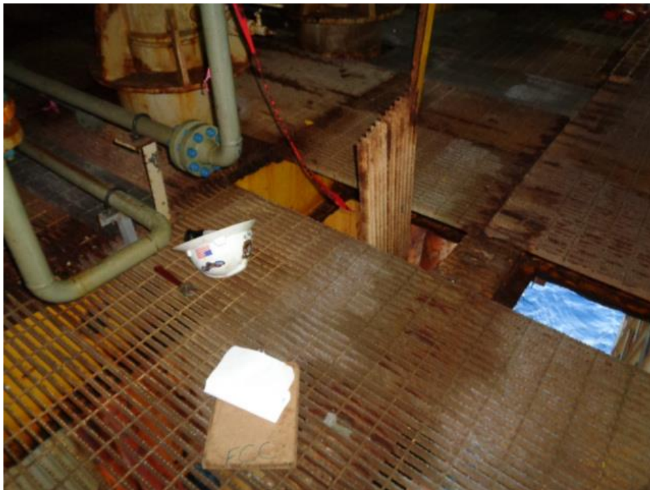
Figure 10- Post-Incident Photograph of Hazardous Grating Section Suspended in Open Hole with Victims Hardhat, Wrench, and Clipboard
