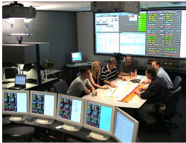
Figure N.4-2 Real Time Operations Center
