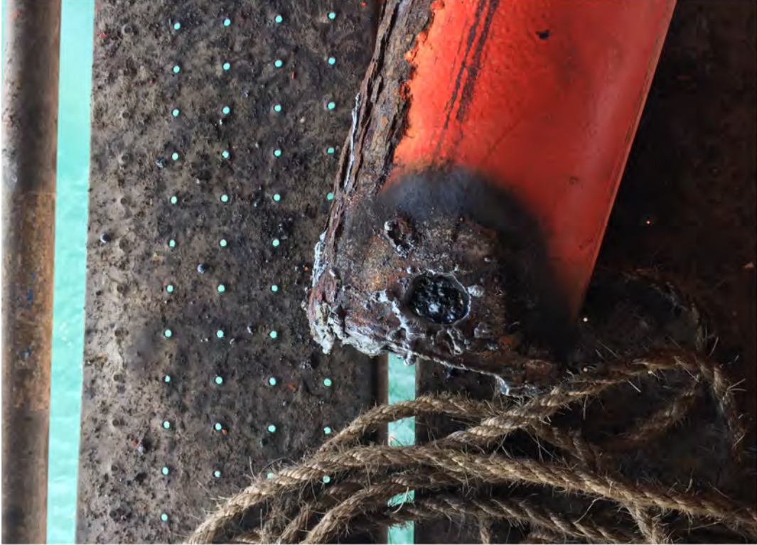
Figure 10: Example of hole torched into the cut sections of pipe
