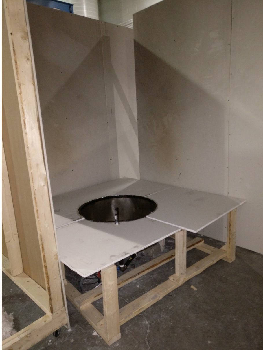
Figure A5. Fuel/water container shown with the full enclosure base in position.
