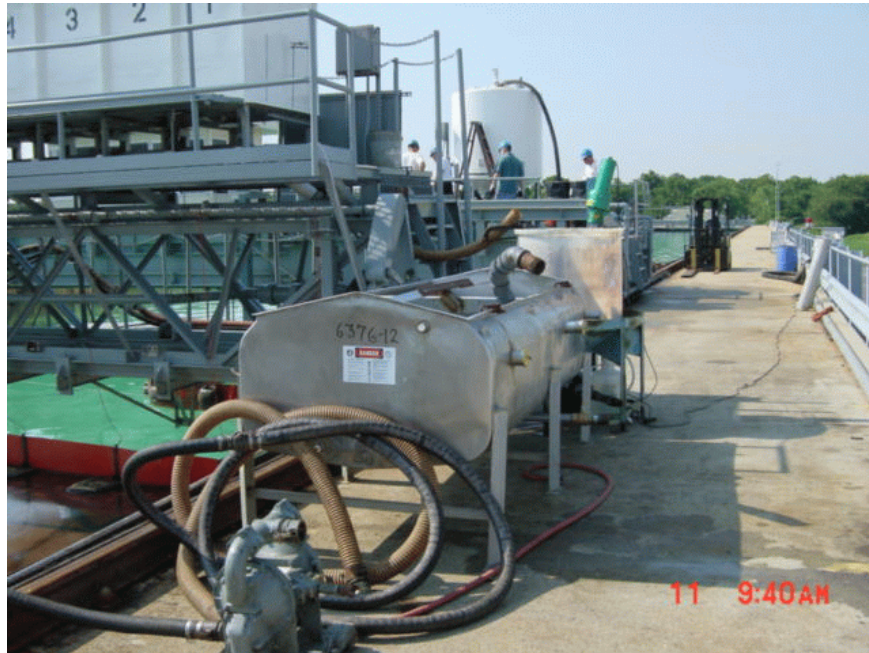
Figure 5 Steel Temporary Holding Tank for Decanted Water
