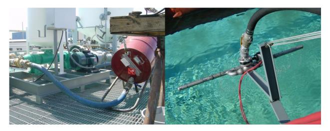
Figure 3. Oil Supply System and Discharge Header
